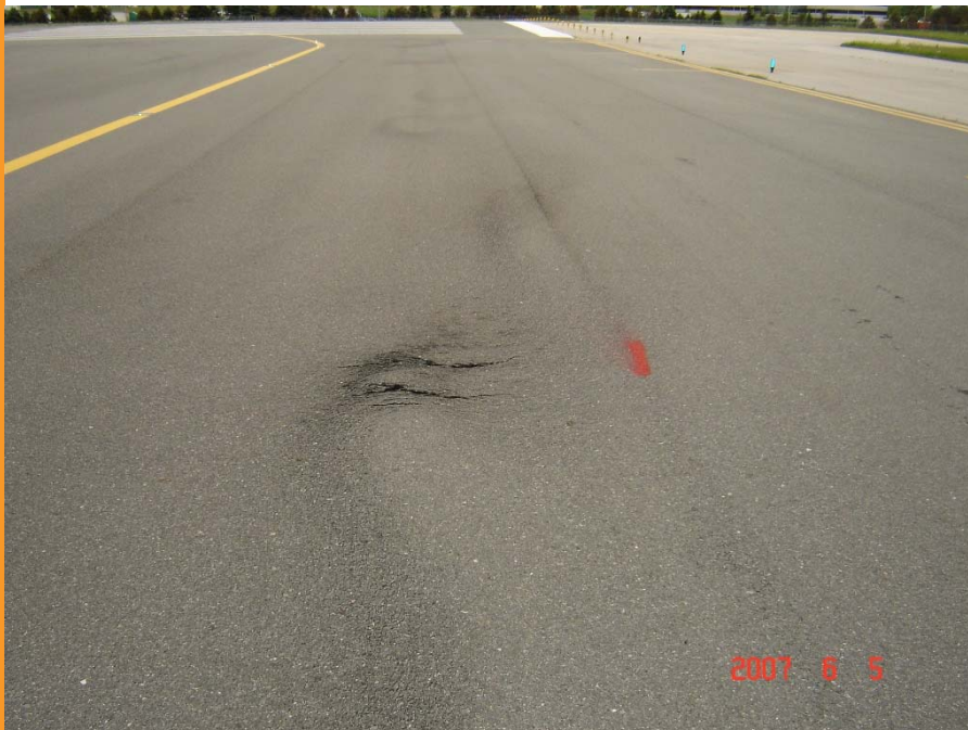
Shoving in asphalt
