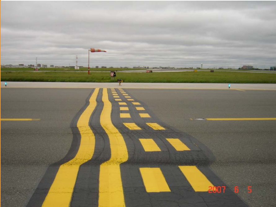
Pavement shoved at the holdline position
