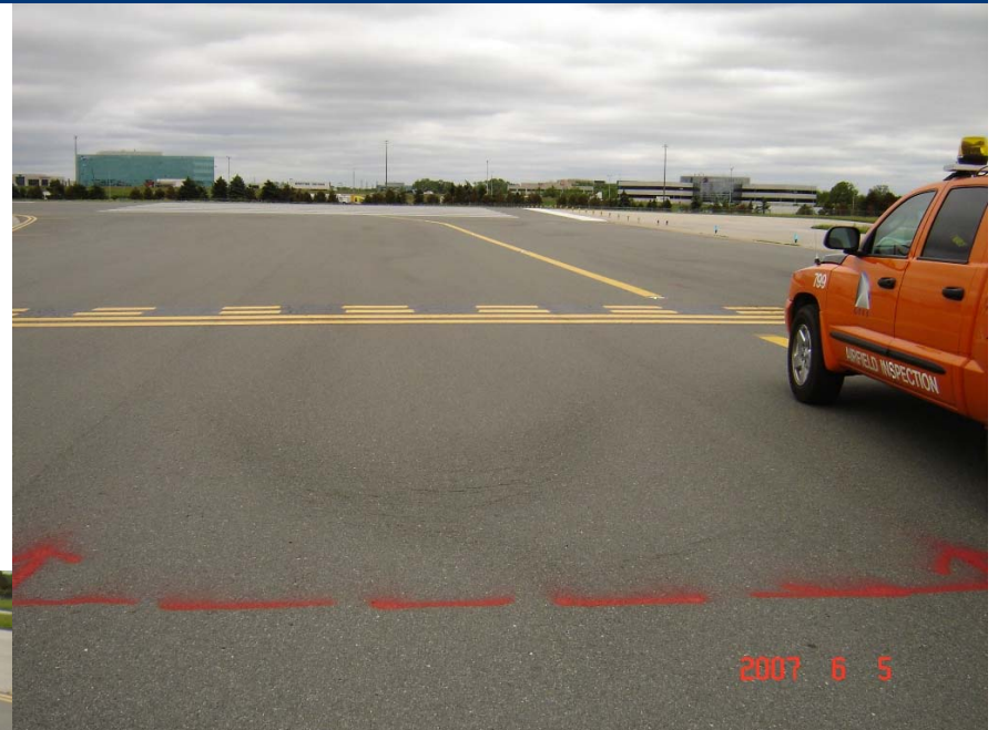
Shoving at locations of heavy braking of aircraft.
