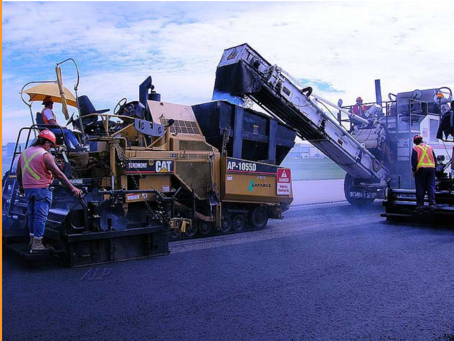
Paving in echelon to eliminate cold joint
