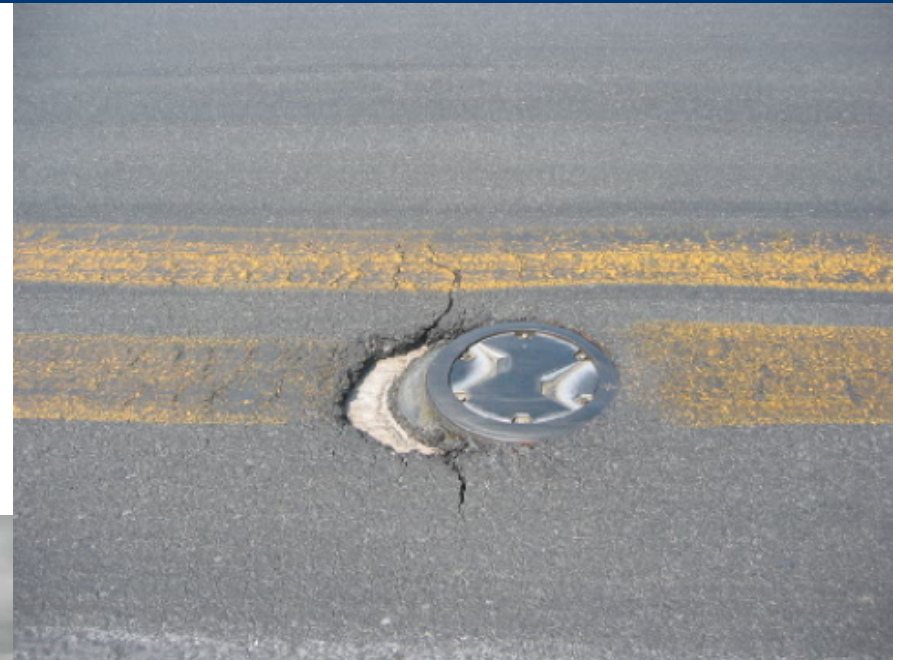
Slippage of asphalt away from the inset light
