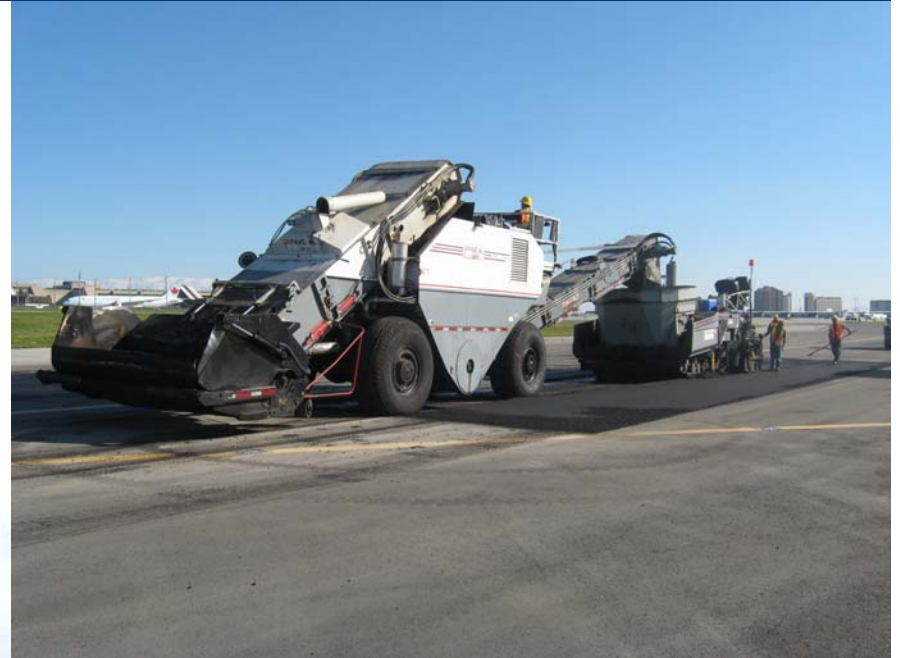
Shuttle buggy to allow paver to run continuously to enhance smoothness and minimize segregation across the mat
